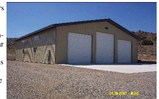
This personal shop building belongs to longtime M&K clients Dick and Doris Atkins. The 50'x60'x14' RV storage shop features three large overhead doors and multiple windows to let in natural light.
