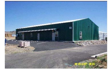
This 50'x90'x14' Vauled Clearspan Truss serves as the new headquarters of M&K Builders.
