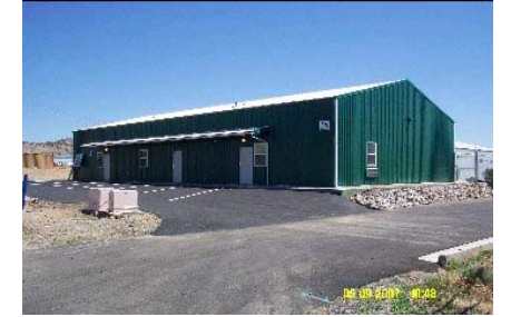
This 50'x90'x14' Vauled Clearspan Truss serves as the new headquarters of M&K Builders.
