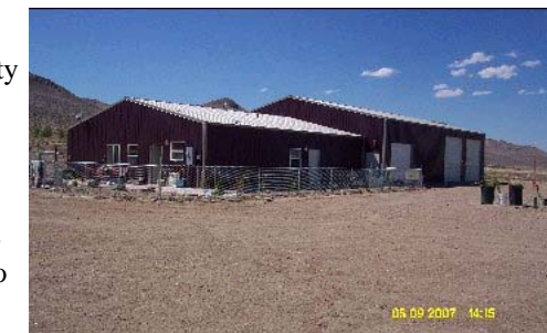
This project featured conjoined buildings, a 40'x42'x10' (living quarters) and a 50'x56'x16' (shop).
